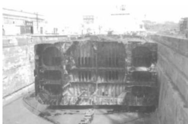
Fig.3 Extent of damage [2.1]
