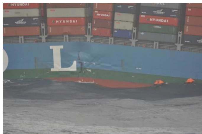
Fig.3 Damage extent (detail)
